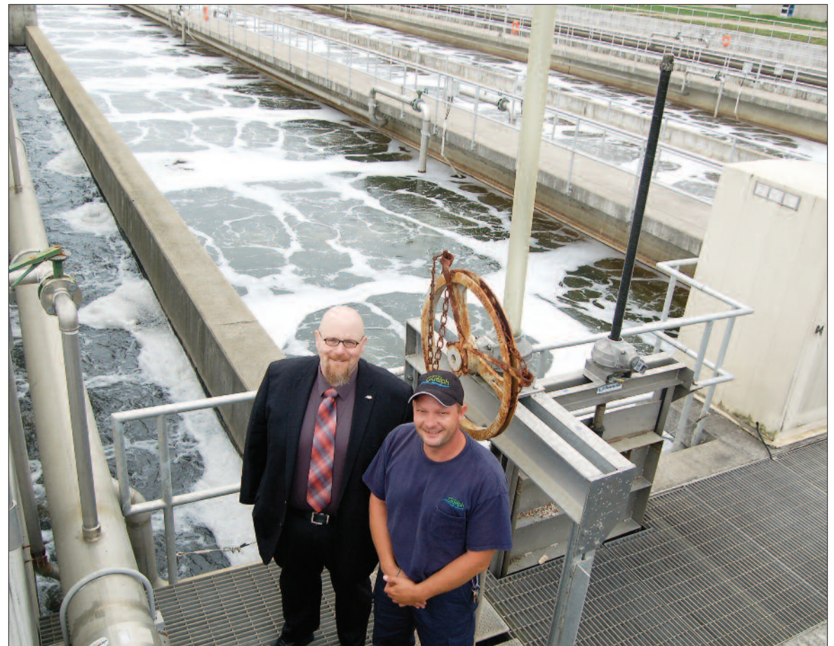
Gerry Atkinson (right), operations lead hand and Cameron Walsh, former manager of Guelph’s wastewater services, during a capacity test of the city’s treatment plant. The test showed the plant can reliably treat more wastewater than it is rated for.
